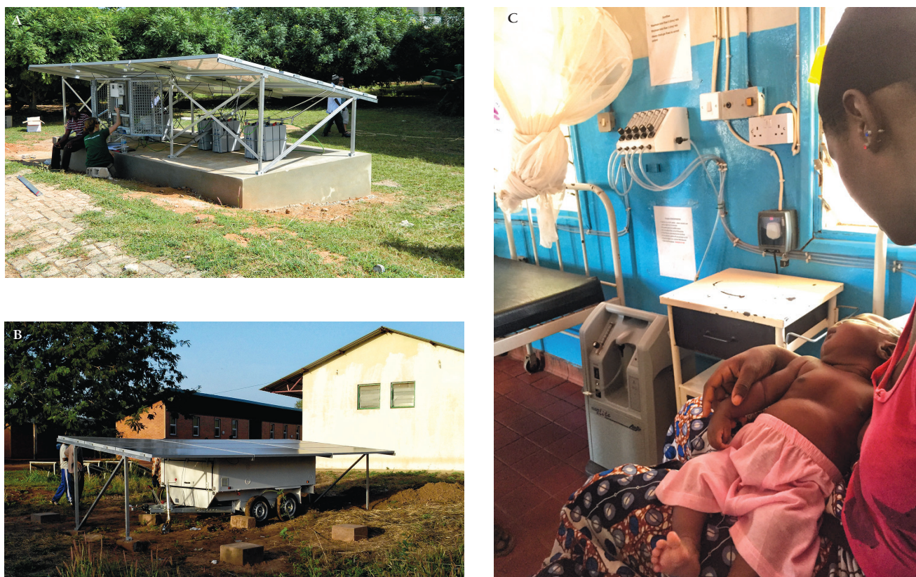
Figure 2. Solar-PS systems in the field. Panel A: Standard Solar-PS systems in situ in AFPRC Hospital, Farafenni, The Gambia. Panel B: Trailer Solar-PS system installed at Soma Health Centre, Soma, The Gambia. *Wheels were subsequently removed and fence erected to deter theft. Panel C: Trailer Solar-PS system supplying oxygen to a child in Soma Health Centre, Soma, The Gambia. *Photograph used with permission of caregiver.
