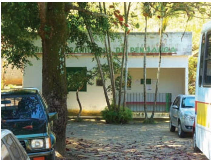
Photo: Unidade Sanitária Rural de Pendanga, Ibiracú (Brazil) – a rural health clinic in Brazil. Via Wikimedia Commons Creative Commons Attribution-Share Alike 3.0 Unported.
